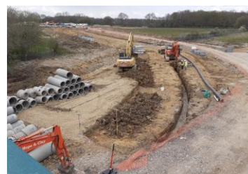
View from the temporary footbridge looking north
