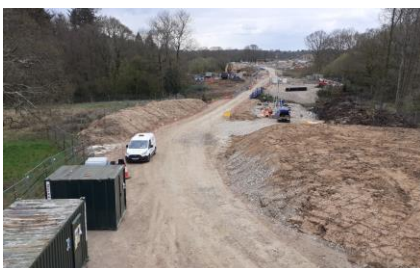
View from the temporary footbridge looking south
